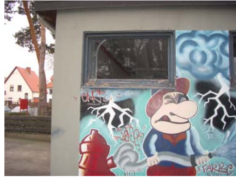
Abb. 14 Holzfenster in Wagenhalle
