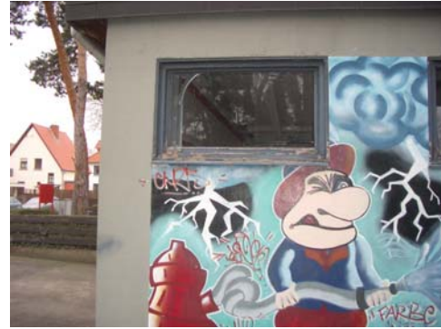
Abb. 14 Holzfenster in Wagenhalle
